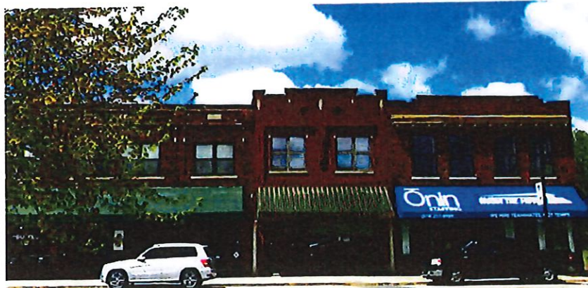
PRECEDENT: Example of the scale and character for the new mixed-use buildings on S. Main Street.
