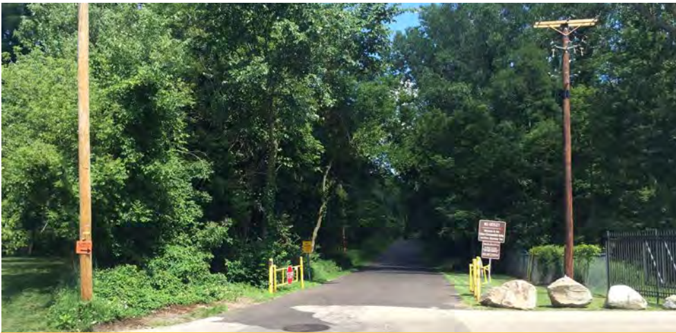
Existing Main Entrance to the EEC
