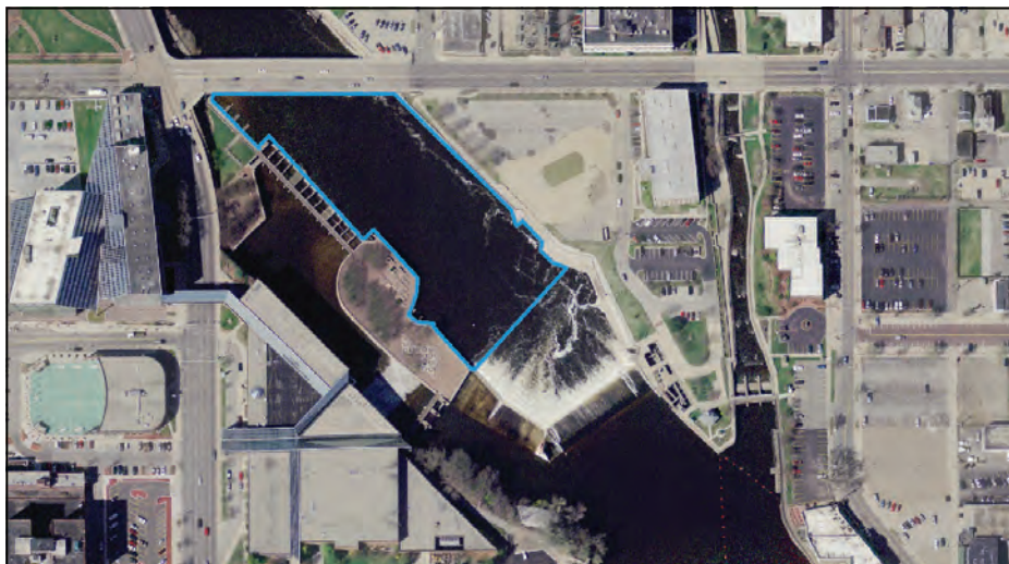
Site #6: St. Joseph River South Bend Dam (B)
