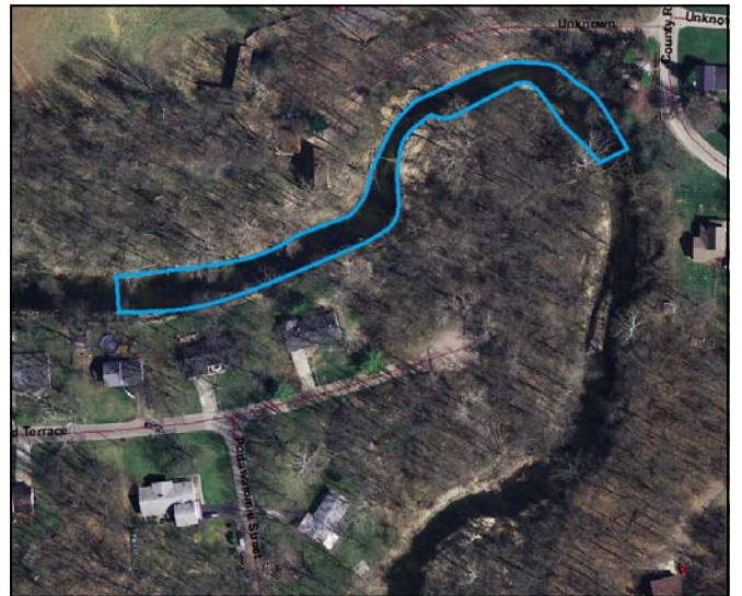
Site #20: Baugo Creek Restoration Site
