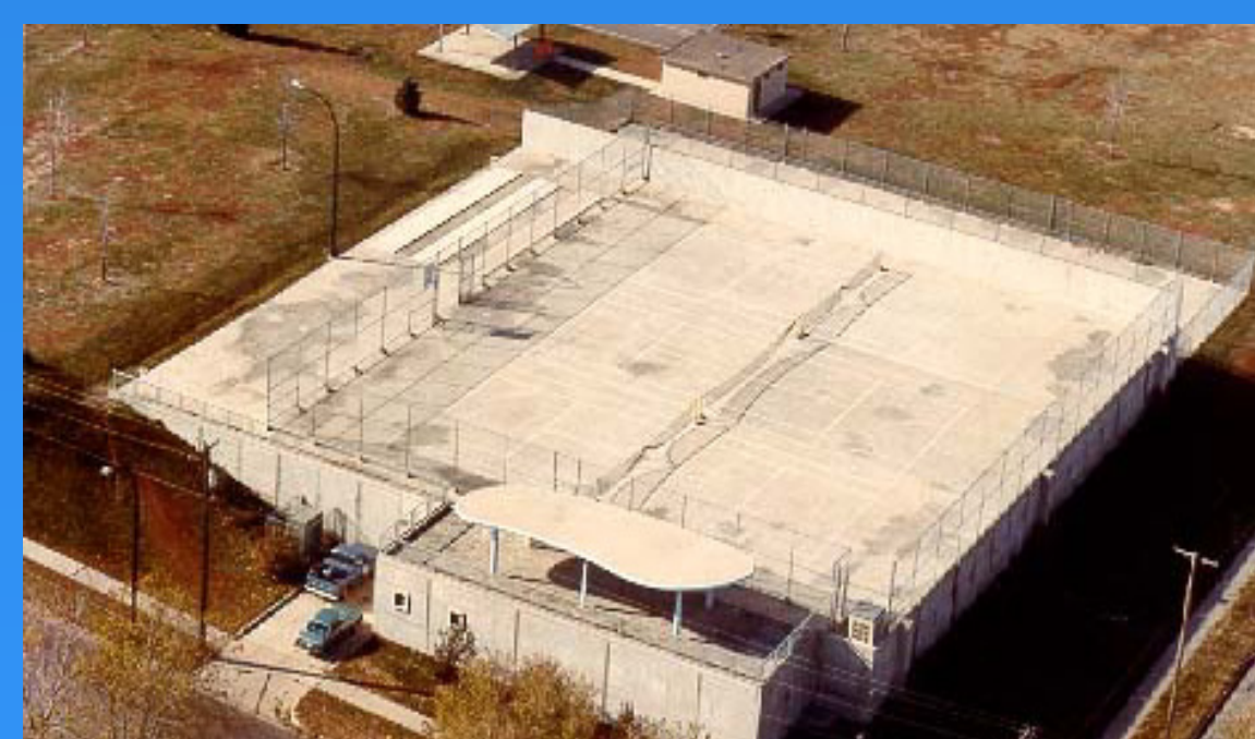
Regional storage tank to capture overflows
