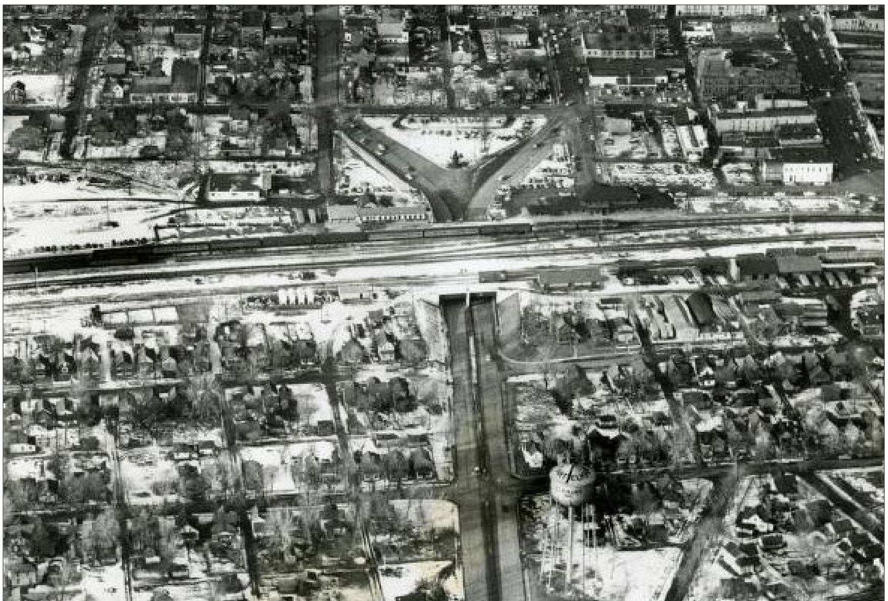
FIGURE 5: Aerial Photo Showing the Impact of the Benham Avenue Underpass, Circa 1963
