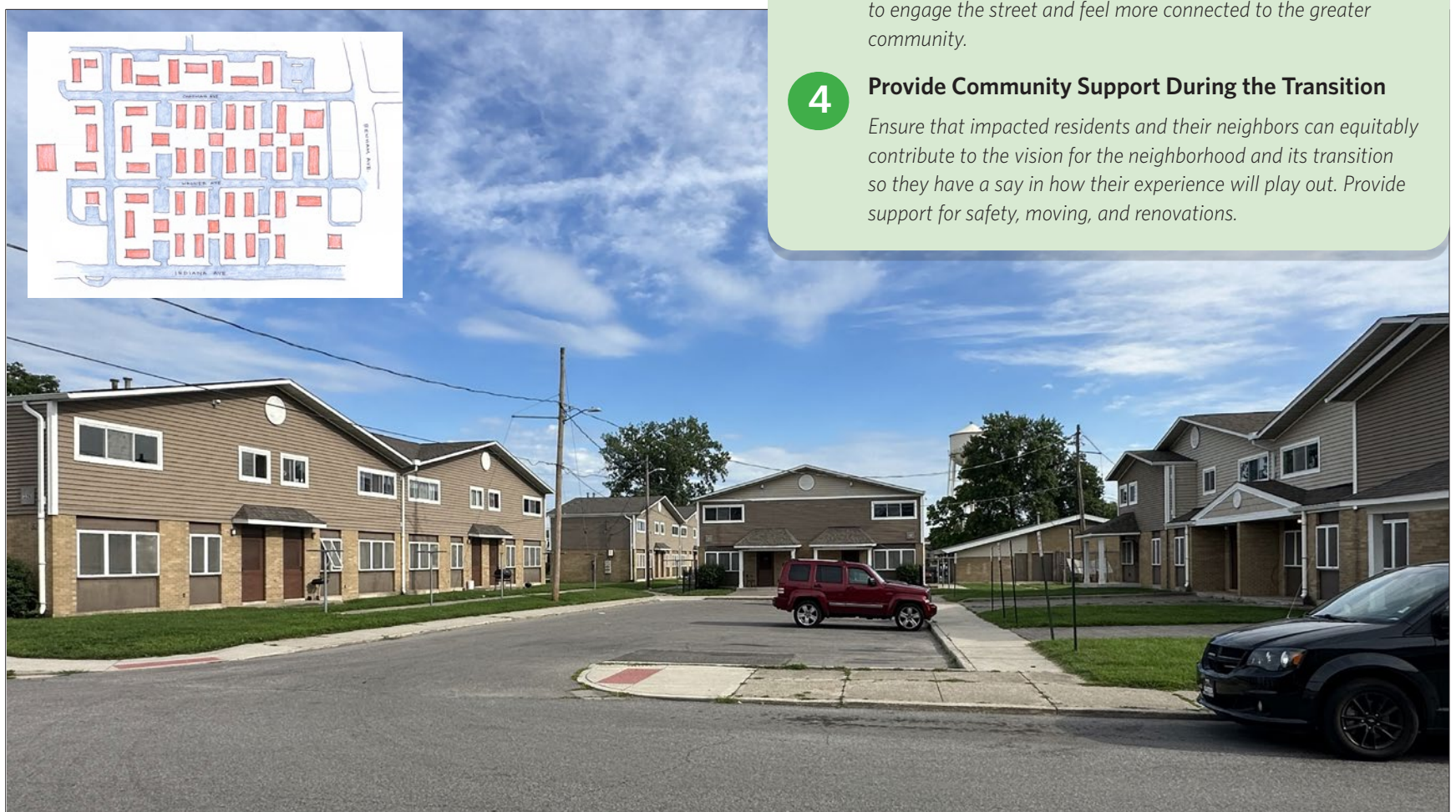
FIGURE 66: Existing Conditions of an Elkhart Housing Authority Parking Pod
